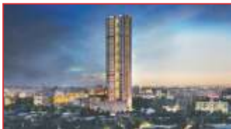
SIDDHA SEA BROOK 247 apartments, 53 Storey Building, Kandivali (West) Mumbai
